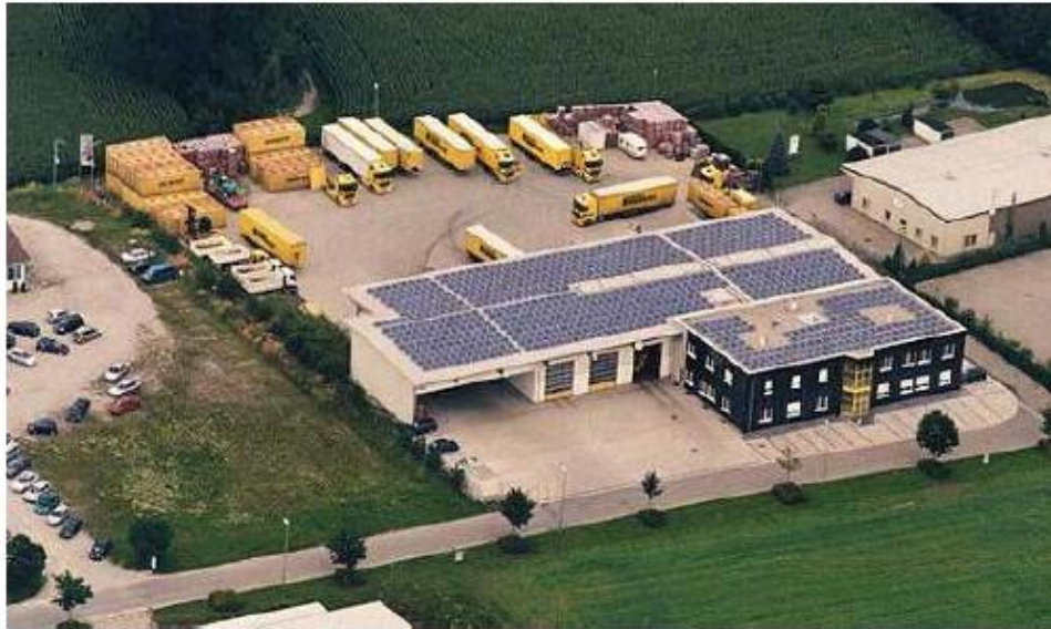
Figure 5: Transportation company Hammerer, Austria, hot water to clean transportation containers for trucks (capacity: 126 \text{ kW}_{\text{th}} ; collector area: 180 \text{ m}^2 ). 6
