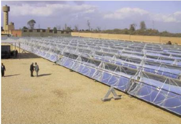
Figure 7: Pharmaceutical Chemicals, Egypt. (capacity 1.33 MW th , collector area (parabolic): 1,900 m 2 ) 6
